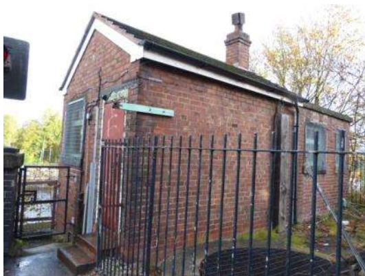
Ancillary Building at south end of bridge
