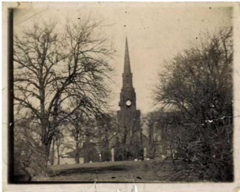
The former Church of St Catherine, 1907 (T.UR.D.283.CAT, Trafford Local Studies Centre)
