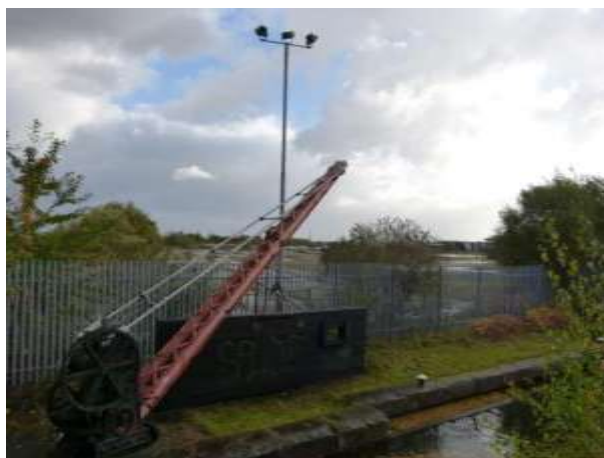
Crane at south end of aqueduct
